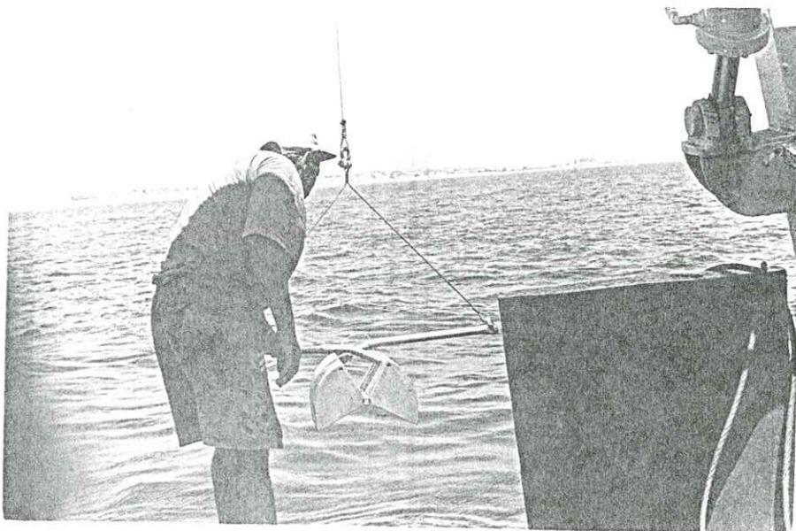
Photo 4: Lowering the grab sampler for taking samples.
