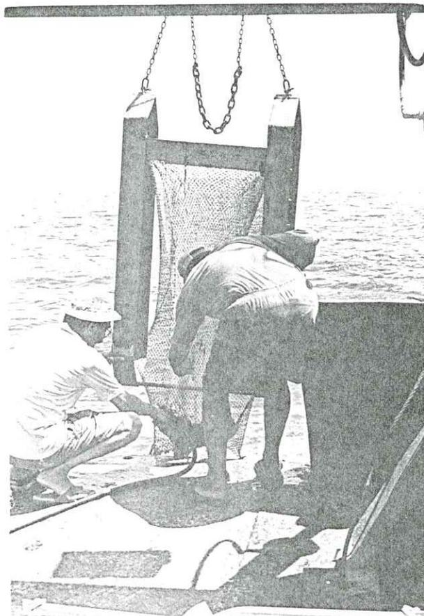
Photo 2: Washing mud and sand from the dredge for subsequent examination
