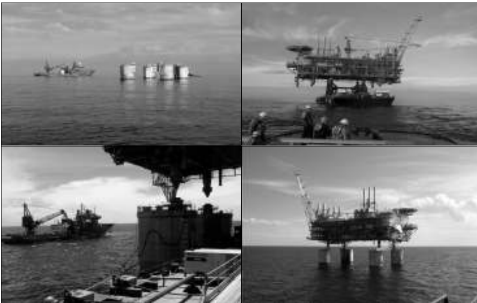
Figure 1 'Floatover' of a gas production facility in the South China Sea.
